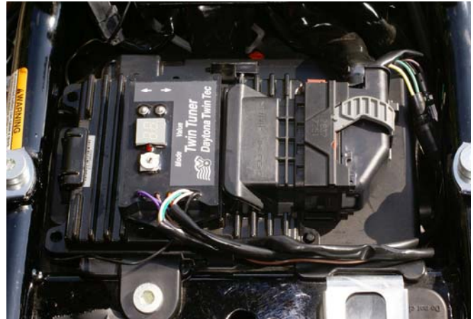
Figure 8 – Completed Twin Tuner Installation
